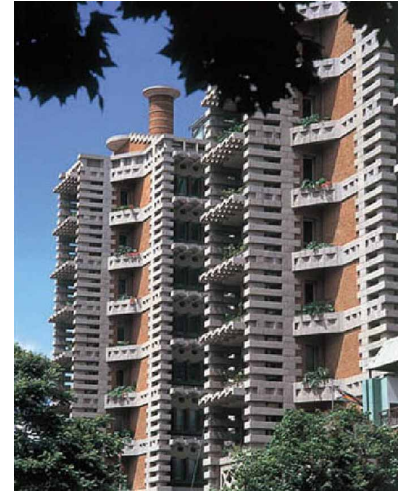
Figure 6: Building in Harare, Zimbabwe, is modelled after termite mounds. Photo by Mike Pearce.
